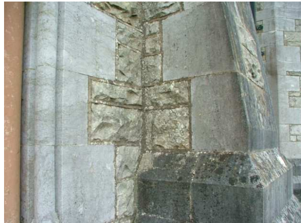
Fig. 25: Hammer-dressed, locally quarried sandstone blockwork to tower elevation (left)
