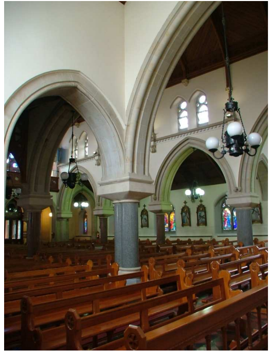
Fig. 19: Gothic arcade of sandstone springing from polished Aberdeen granite columns (right)
