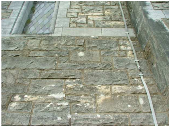
Fig. 25: Hammer-dressed, locally quarried sandstone blockwork to tower elevation (left)
