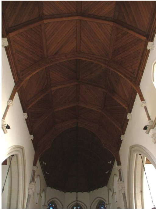
Fig. 18: Pitch-pine panelled ceiling to nave and apse (left)
