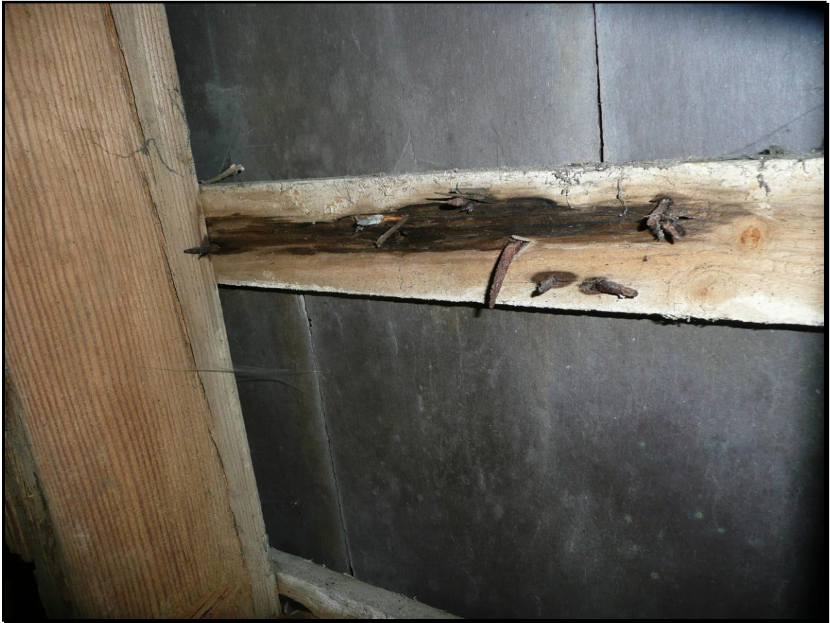
Corroded slate fixings and decayed batten
