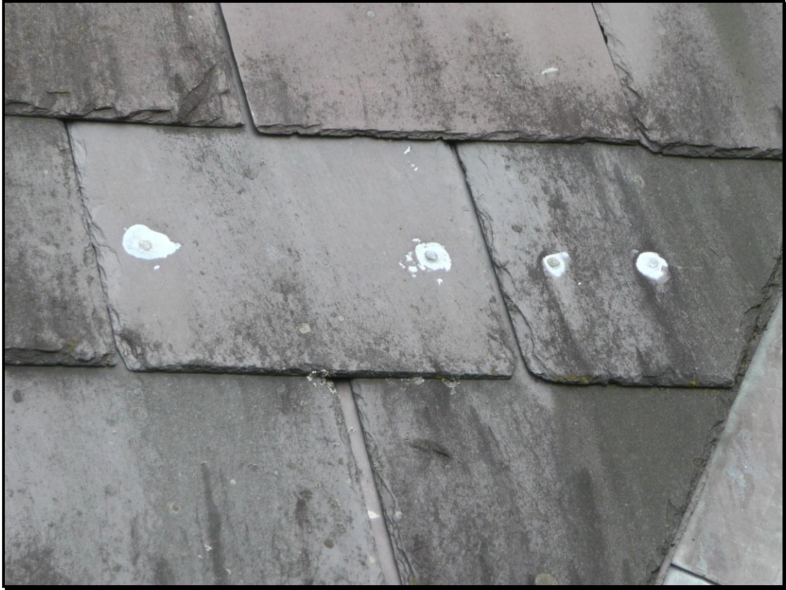
Slates repaired with nails and sealant
