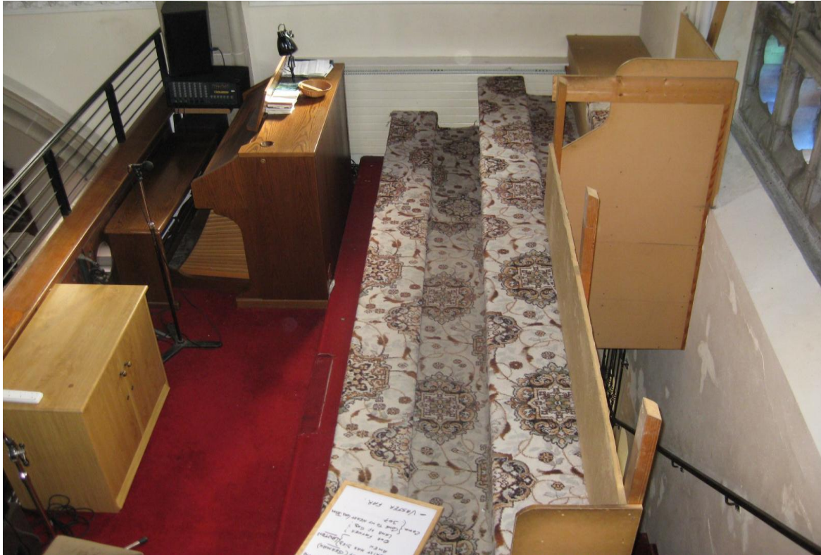
Existing First Floor Gallery – Inadequate/Unsafe Railings
