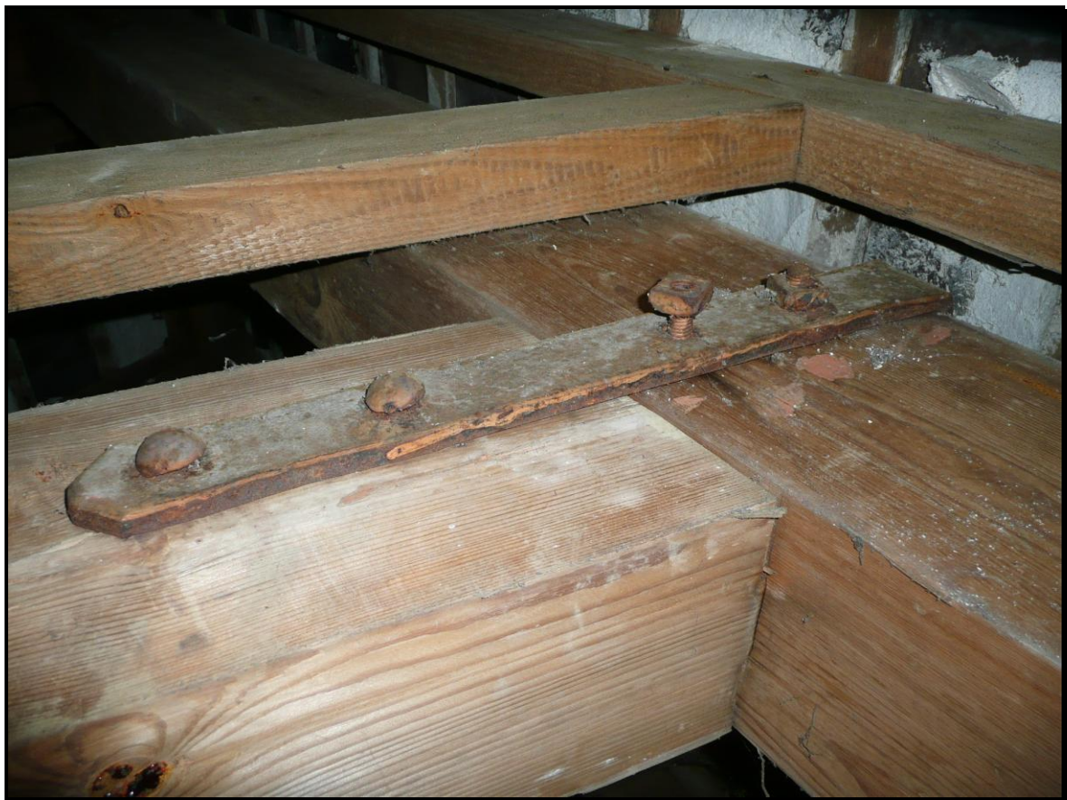
Corrosion and loose bolts in truss straps
