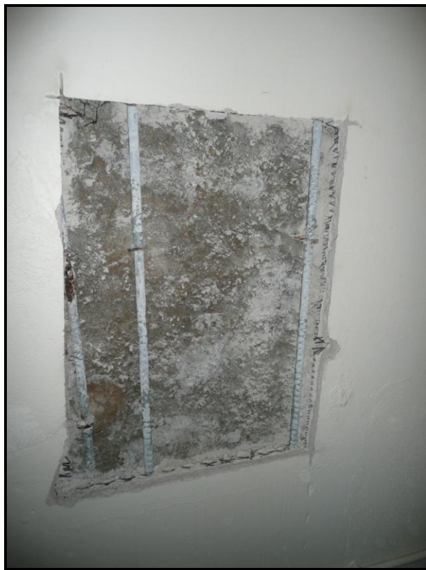
Dry-lined plaster to internal face of rear (west) wall
