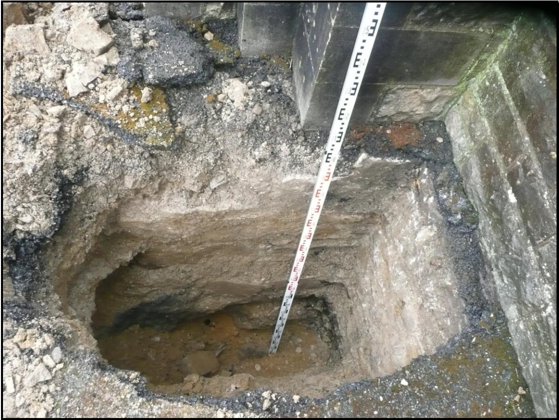
Trial pit excavated at northern corner of belltower
