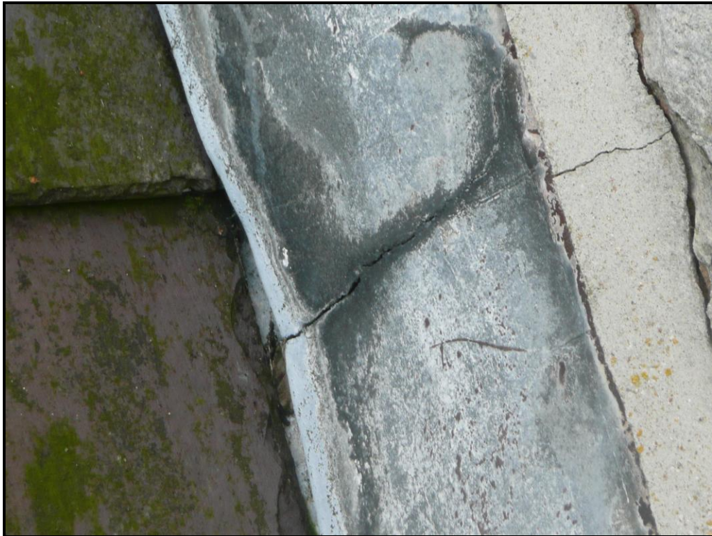
Cracked lead flashing to south eastern elevation of nave
