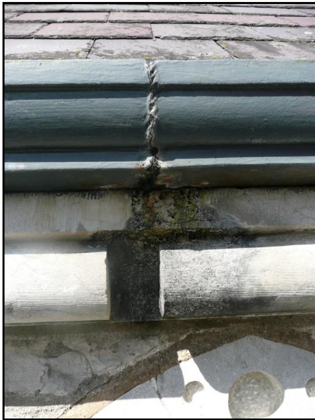
Leak at joint in gutter
